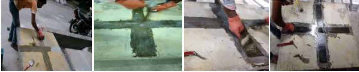
Figure 3: Application of BFRP Sheets
