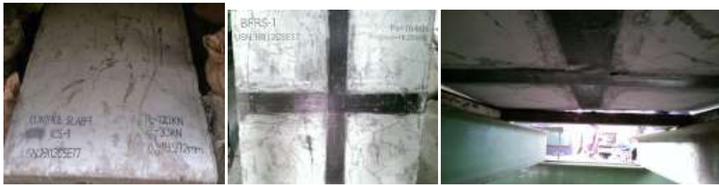
Figure 5: Crack pattern of control slab and retrofitted slab, Mode of failure: De-bonding of BFRP
